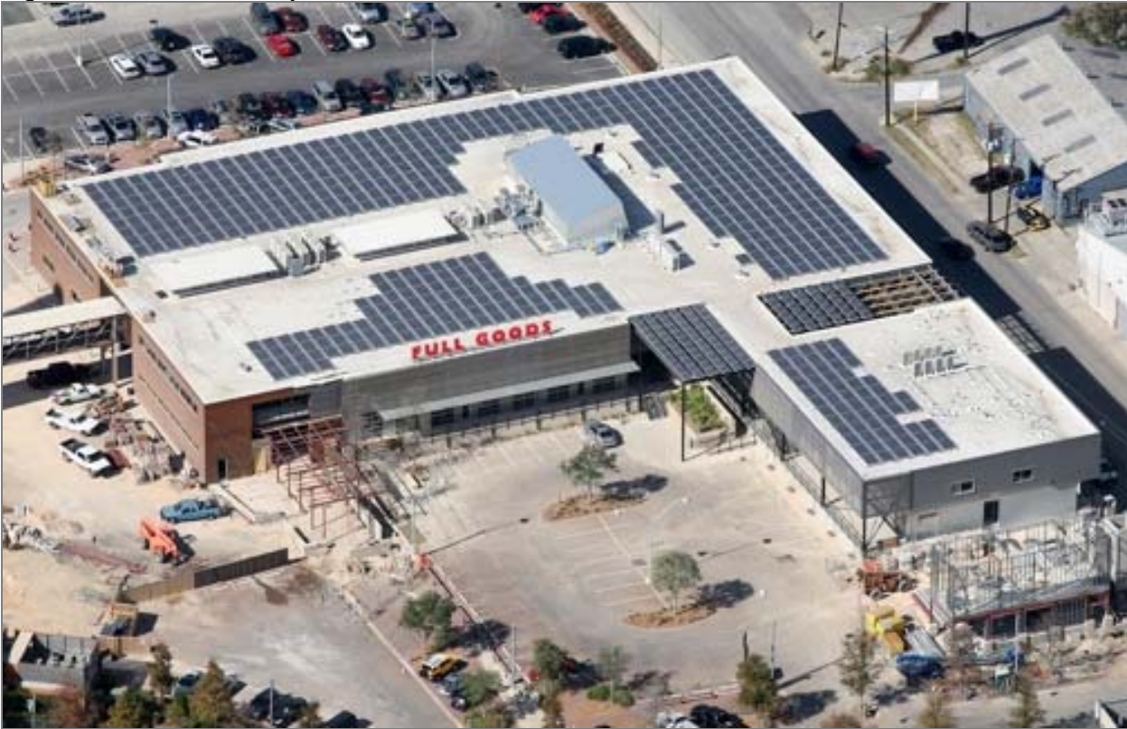
Figure 5-3: Pearl Brewery Solar Insulation
