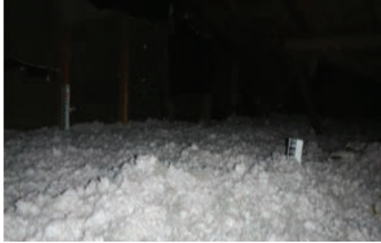
After - Insulation added to create thermal barrier
