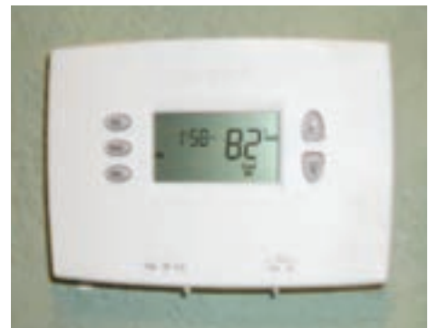
After – Digital Programmable Thermostat to set temperature to maximize energy efficiency
